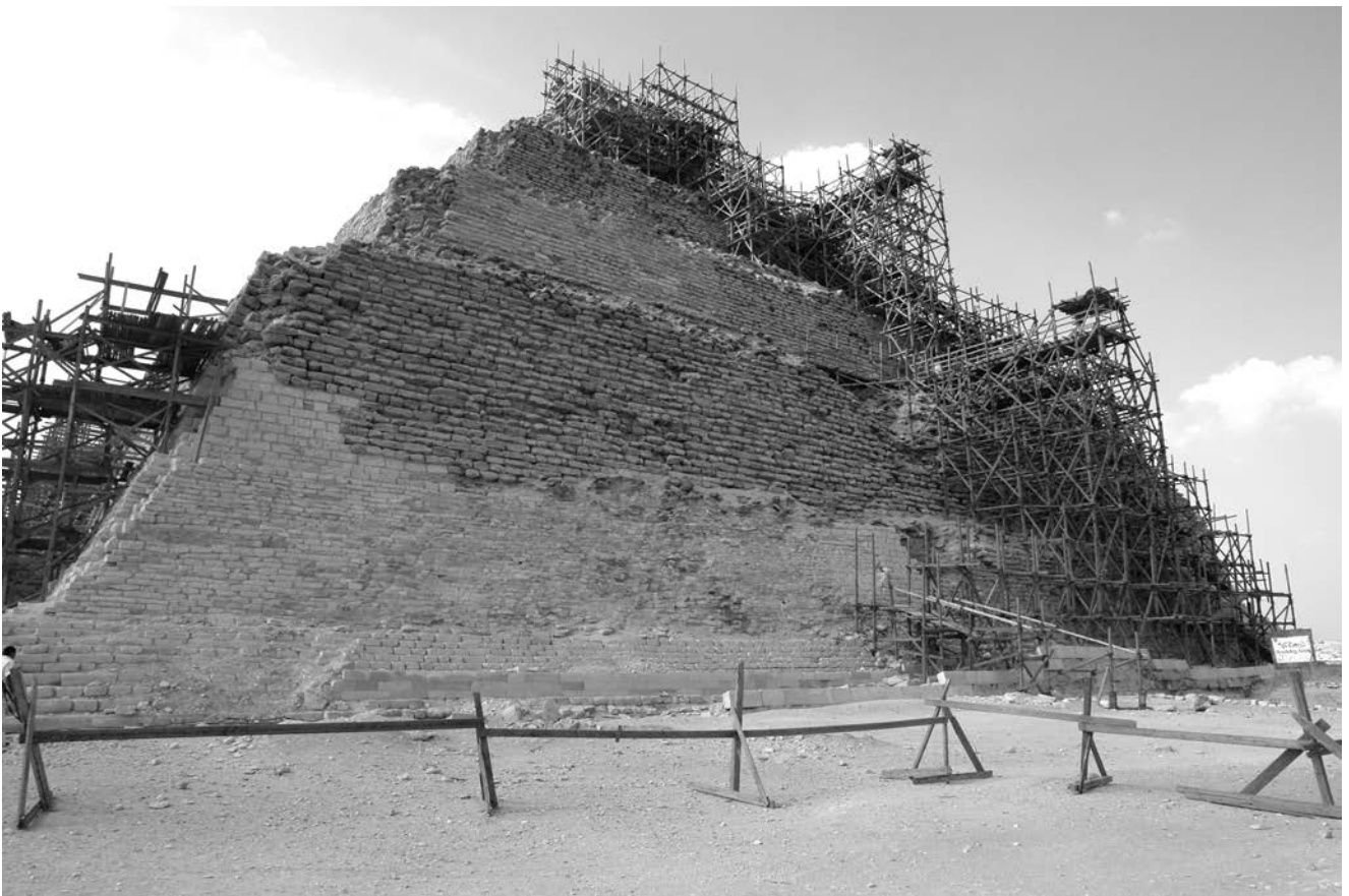
Fig. 5. Step Pyramid’s reconstruction process. Eastern facade in the year 2012.
