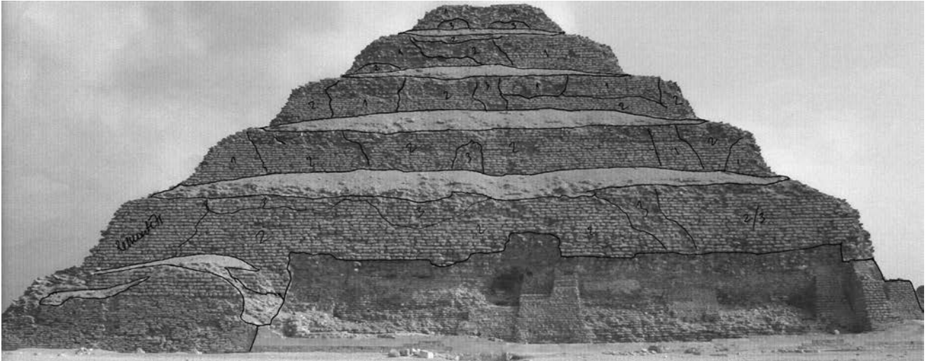
Fig. 4. Schematic depiction of possible construction stages of the Step Pyramid, characterising various quality of the stone material used (different quality material is marked as “1”, “2”, and 3”).
