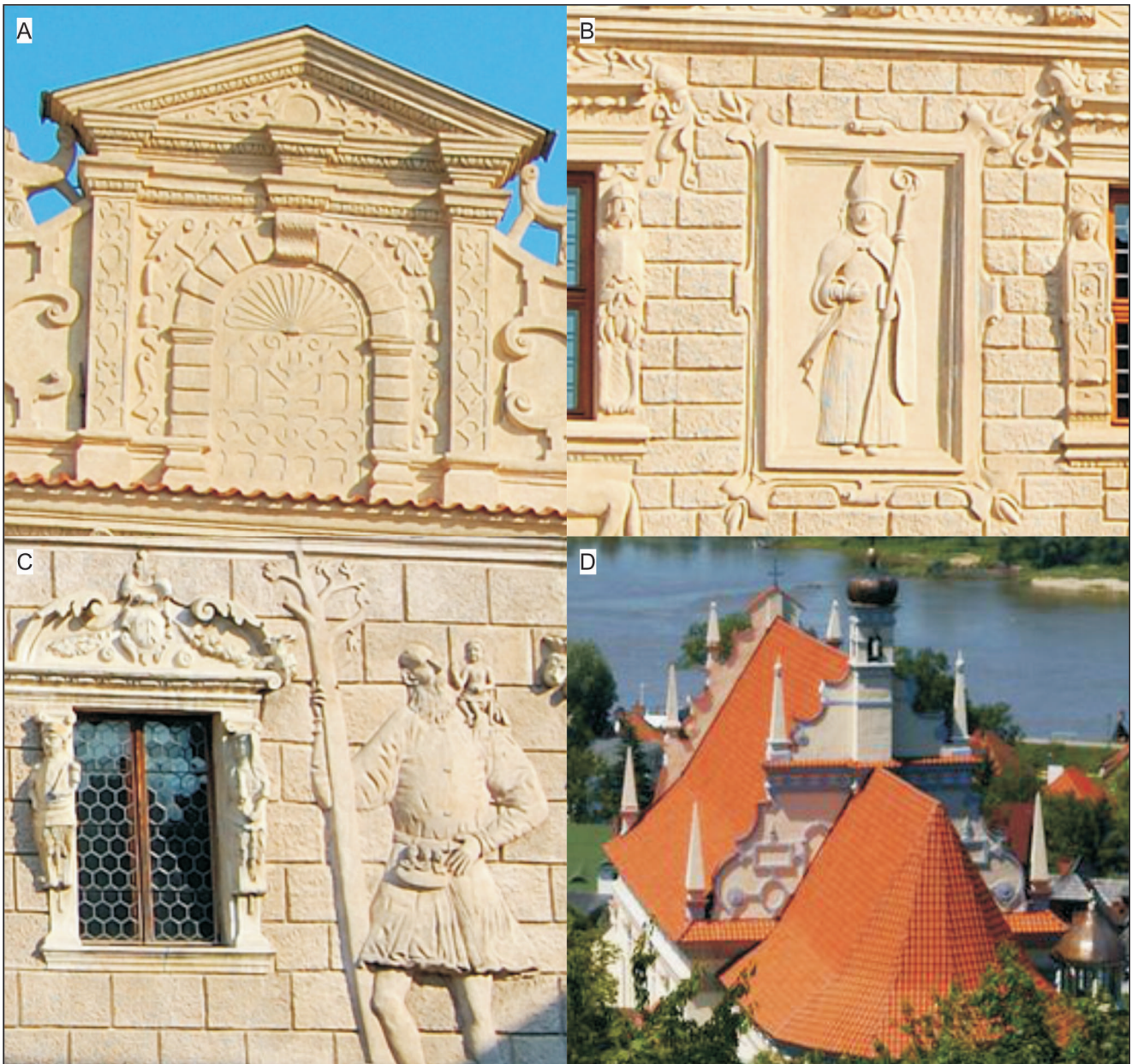
Fig. 2. A, B, C – Ornamental facades of Przybyla brothers' town houses at St. Christopher Street (ca.1615); D – church of St. John the Baptist (1586–1589).
